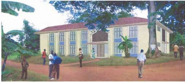
ICMI's building project at Uganda Christian University is now underway.
